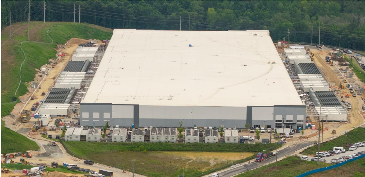
Figure 5: Serverfarm datacenter adjacent to VoltaGrid with 36 diesel engines (white units flanking either side of the building). Images © Michael A. Schwarz.
