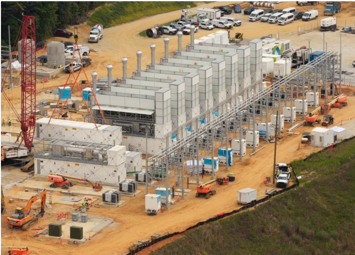
Figures 2 & 3: June 25 images showing eight engines completed and three under construction. Images © Michael A. Schwarz
