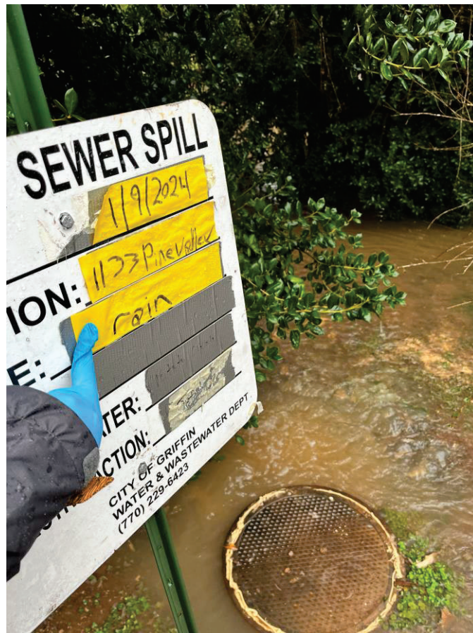
Figure No. 2: Manhole No. 1
